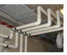
more than 1.25 kilometers from the shore to the lake bottom. To ensure safety and reliability, the chemical feed system that transports the ferrous chloride diluted with carrier water is double contained to prevent any possible leaks or spills.
