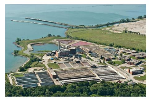
Originally built in the late 1950s to handle an average flow of 2 million gallons per day (mgd), the G.E. Booth (Lakeview) Wastewater Treatment Plant (WWTP) is a key facility for the Region of Peel. In 2009, the facility underwent a \$260 million expansion to treat 137 mgd from the more than 1.3 million residents and 90,000 commercial businesses in the eastern section of Mississauga, Brampton, Bolton, and Caledon East.
