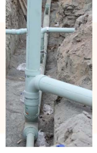
The easy-to-use guided Enfield machine allows for ease of installation; the fittings have an outside marker for the metal clamps and a stopper embedded inside the fittings, so we don't need to measure how far the pipe needs to go in.
