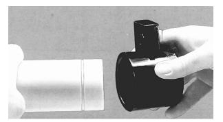
2. Verify the grooving tool is sharp. Cut the pipe to the desired length using a tubing cutter fitted with a wheel designed for plastic pipe. A handsaw and miter box may also be used. Ensure pipe ends are square and trimmed free of burrs.
