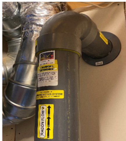
Figure 3: RadonX system utilized for a Level-3: Active System radon mitigation system
