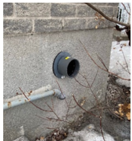
Figure 3: RadonX system utilized for a Level-3: Active System radon mitigation system
