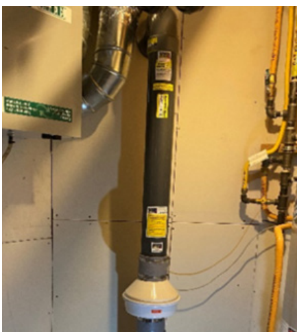
Figure 3: RadonX system utilized for a Level-3: Active System radon mitigation system
