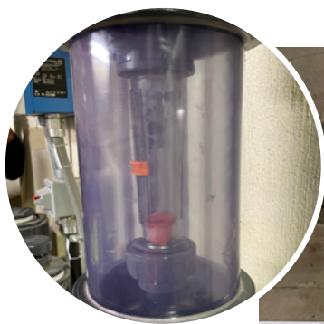
A clear containment system allows for easy detection of leaks
