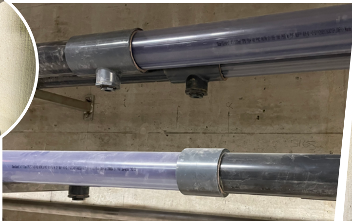
A clear containment system allows for easy detection of leaks
