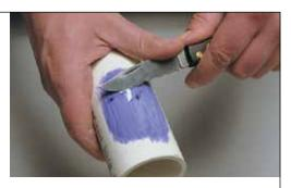
scratch or scrape a few thousandths of an inch of the primed surfaces away.
