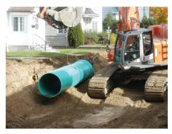
IPEX Group says its Ring-Tite brand pipe is made with a high-strength, high-impact PVC compound for municipal sewer systems to stop threats like cracking, leaking and corrosion. The company expects U.S. infrastructure needs to boost demand for plastic pipe in 2021.
