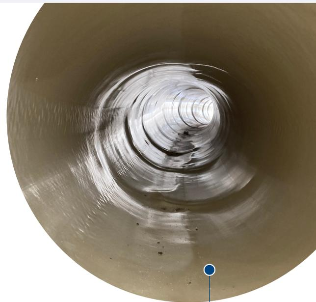
Fully functional pipe after the existing clay pipe is relined with NovaForm PVC liner
