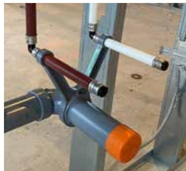
System XFR Water Line Installation
