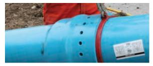
4 Once the holes on the bell are aligned with the inner groove, line up the pins on the external half ring with the holes in the bell so that the half ring covers either the left or right side of the pipe.
