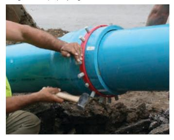
6 Check to make sure all of the pins are fully inserted before starting the next joint.
