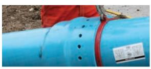
4 Once the holes on the bell are aligned with the inner groove, line up the pins on the external half ring with the holes in the bell so that the half ring covers either the left or right side of the pipe.
