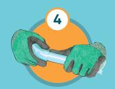
**DRY-FITTING.** Before applying primer or solvent cement, test all connections (pipes, fittings and accessories) to confirm a proper interference fit exists.
