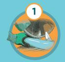
CUTTING THE PIPE. It is important to cut the pipe squarely. A square cut provides the surface of the pipe with the maximum bonding area. Pipe can be easily cut with a wheel-type plastic tubing cutter, chop saw or fine toothed saw. Do not use reciprocating saw.
