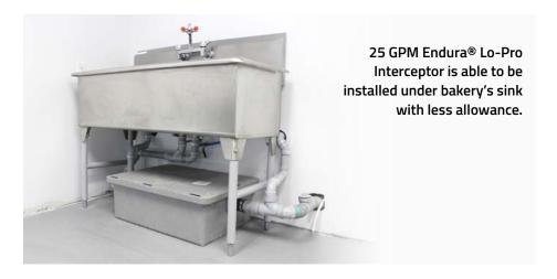
"Rather than sliding the baffles up vertically to remove them, the Endura Lo-PRO's unique design allows you to slide them up vertically about halfway then tilt it about 45 degrees to remove them. This allowed us to reduce the required overhead clearance to only 5 inches."
