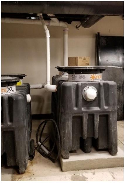
Two Endura® XL100 Grease Interceptors were installed in the basement of Half-Shell Oyster House
