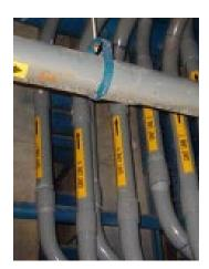
Duraplus<sup>™</sup> Industrial ABS is 1/4th the weight of steel, making it easier to transport on site. Duraplus Industrial ABS is joined by a solvent cement system, so special equipment is not required.
