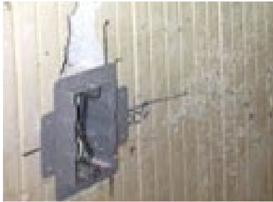
More than 700 electrical boxes were needed throughout the new hotel for power and data connections
