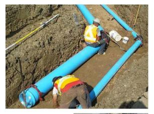
completed and the new watermain commissioned, a 4" gas line was being installed and the contractor drilled directly through the center of the new 12" watermain.
