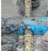
"I was really surprised that the Bionax PVCO held together. Had this had been a C900 pipe the damage would have been much more extensive with a bigger mess to clean up". Smith's crew worked fast as they cut out a 6 foot section and tied in the repair with two couplings. "The repair was clean, and easy to complete as the damage was contained within inches of the affected area".
