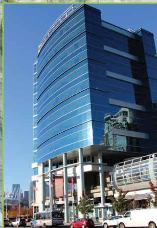
Vancity Goes Green with HVAC
