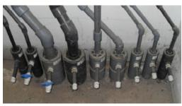
The IPEX Guardian<sup>™</sup> Vinyl double containment system was required for underground runs, which transitioned to IPEX single wall PVC and Corzan CPVC inside the facility.
