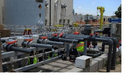
IPEX Corzan® CPVC pipe, valves and fittings are used in areas transporting highly-corrosive chemicals.
