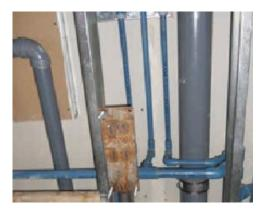
System XFR has less potential to form condensation, which can ultimately reduce or eliminate the cost of adding insulation.
