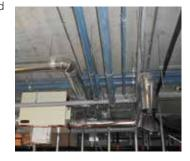
Montpellier. On each floor, it branches off to the apartment units where it transitions over to traditional PEX pipe. Because each unit includes its own hot water heater, AquaRise is used for cold potable water distribution only. The system was designed by Desjardins Expert Conseil (www. genieconseil.com), the mechanical and electrical engineer for the project who has been installing IPEX products for many years.
