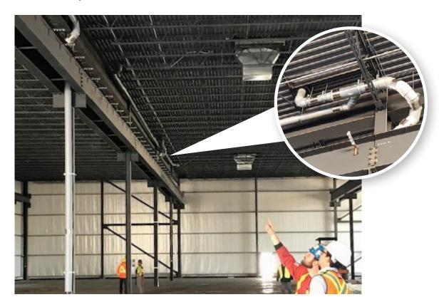
n spring 2019, a new Windsor warehouse for Erie Architectural Products was under construction. Bryant Heating, Air Conditioning & Plumbing used System 15® PVC in 6", 8", and 10" diameters to install the rainwater leaders.
