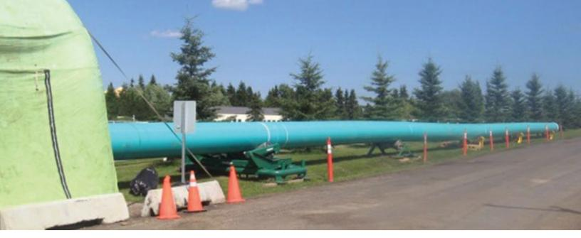
Fusible Brute PCV pipe ends and fusion machinery are sheltered during the installation
