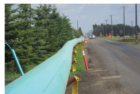
"I ended up fusing about 40 joints for this project, completing about five joints a day. The warmer weather meant more cooling time for the joints, but it was a lot easier than needing to bring in shelter and heat," said Roger Zwaan, the fusion technician with Clean Harbors Direction Boring. "Because the directional boring process was taking place later, I did about 300 meters in June and then came back and finished up the remaining joints about a week before the pull date in September."
