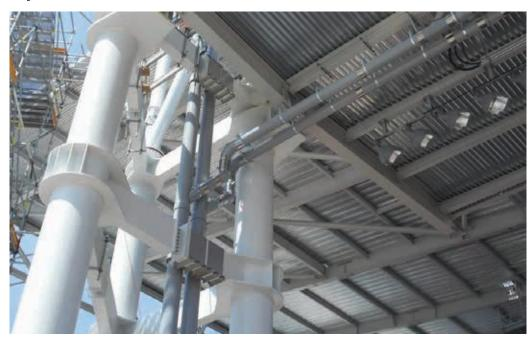
IPEX System 15® DWV was used to drain water from the canopies into the existing storm water system
