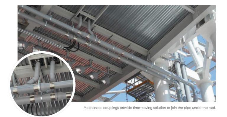
the pipe instead of solvent welding. Mechanical couplings were a great alternative to solvent welding when working at heights in a scissor lift or bucket as was necessary on this project.
