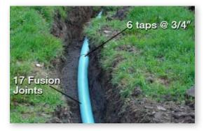
Photo 2: Six 3/4" taps and seventeen fusion joints were installed.
