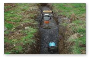
Photo 3: Bedded and covered pipe was capped, filled and pressurized.
