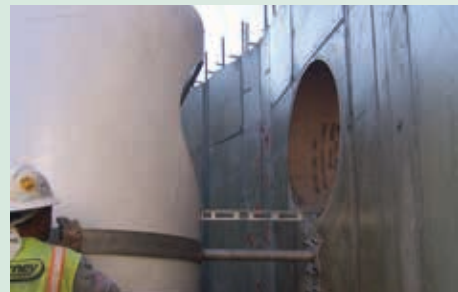
Strapping detail on Vortex unit, Buckeye, Arizona.
