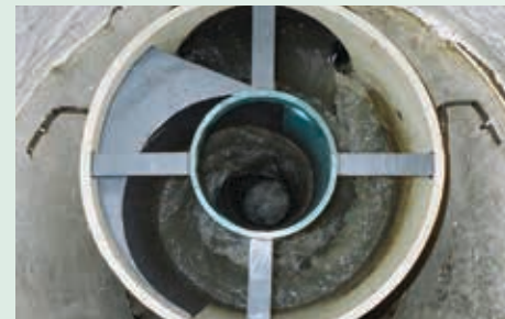
Vortex Flow Insert reducing H 2 S concentration levels, Camden County, New Jersey.
