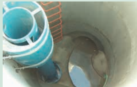
Second effluent line at bottom, benching from the EDP to direct flow, Sarnia, Ontario.
