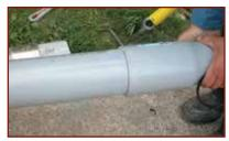
Push the locking spline into the insertion hole at the top of the joint and feed it into the opening. When the spline is completely inserted into the pipe's inner groove, it will lock the lengths together.
